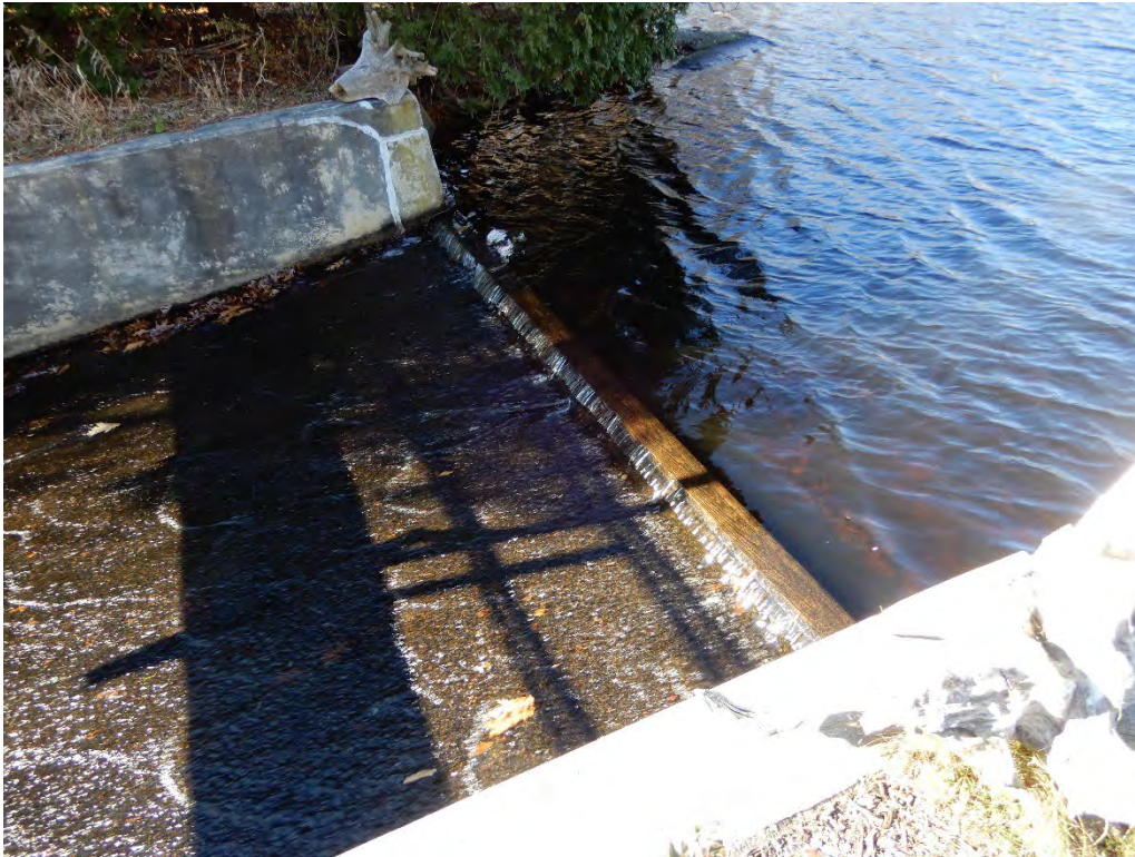
Photo 13 – An overview of the spillway weir, seen from its left side.
