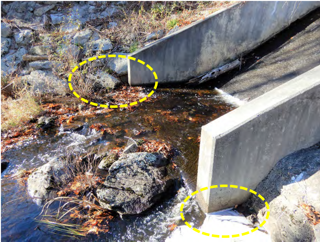
Photo 19 – Although submerged at the time of inspection, this photo depicts the location of the spillway toe drain discharge at the base of the right side training wall (upper center of photo) and the low level outlet pipe discharge at the lower right of the photo.
