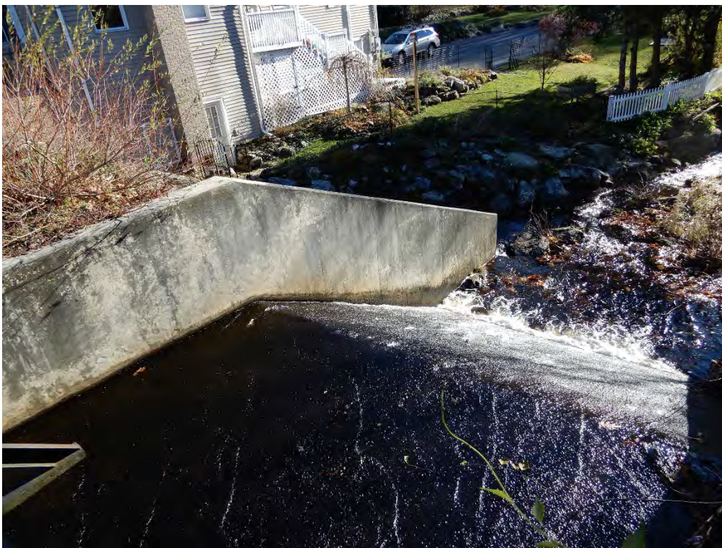
Photo 12a – The lower end section of the left side spillway training wall.
