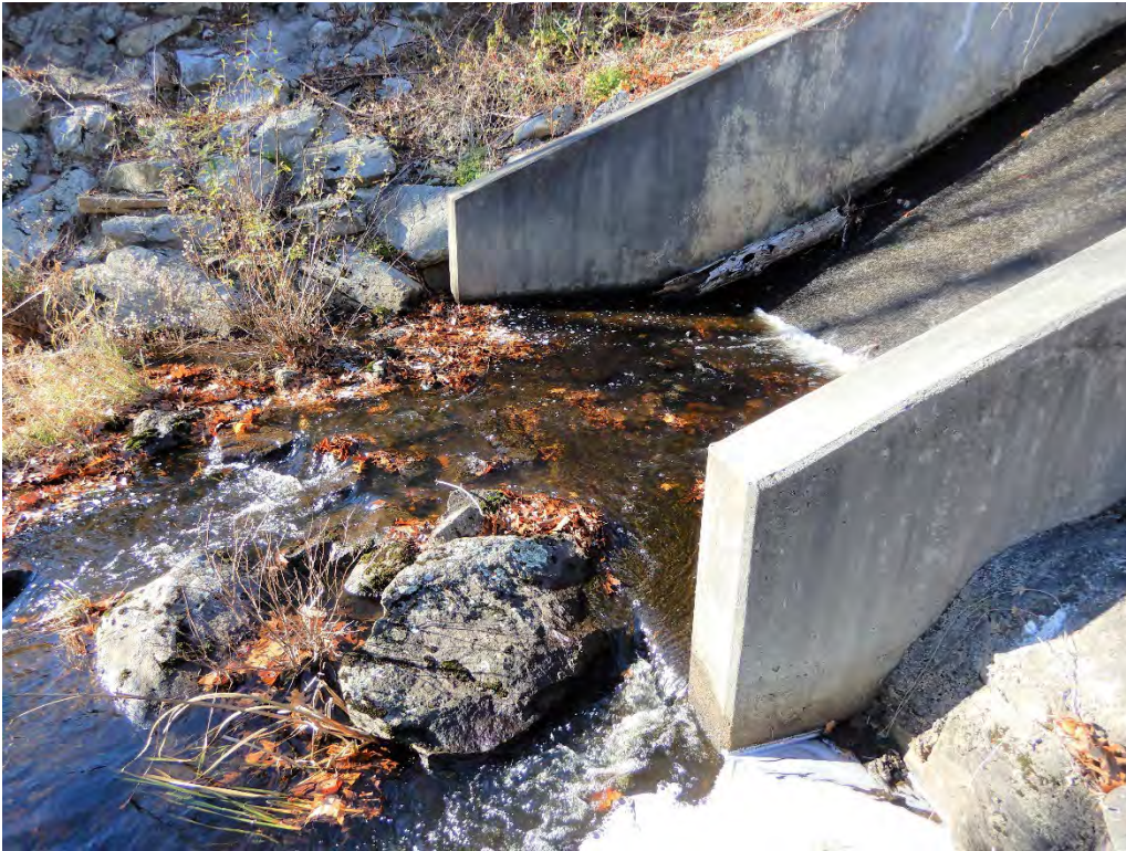
Photo 14b – Another view of the stilling basin at the downstream toe of the spillway.
