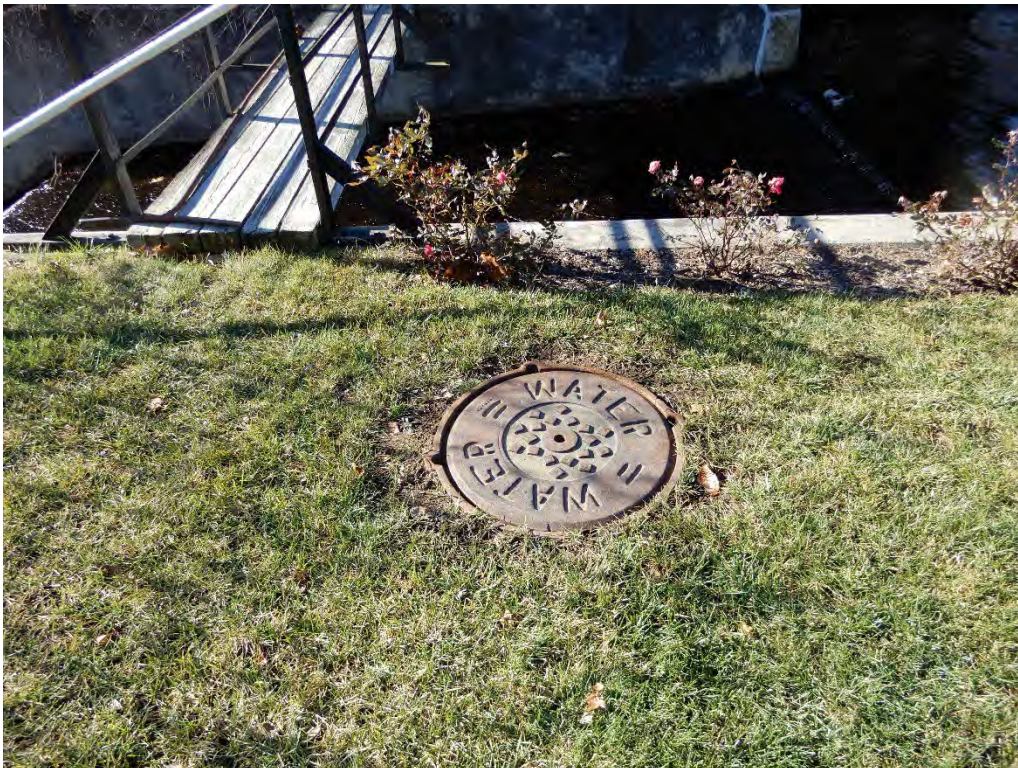
Photo 16 – An exterior view of the manhole housing the gate valve and control stem for the low level outlet.
