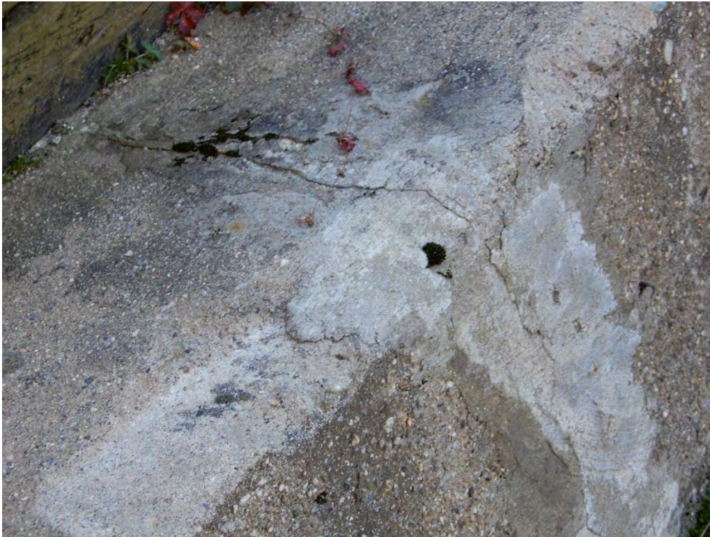
Photo 21c – A closeup of the area shown in the previous photo with an example of the minor cracking patterns developing in a previously patched area.
