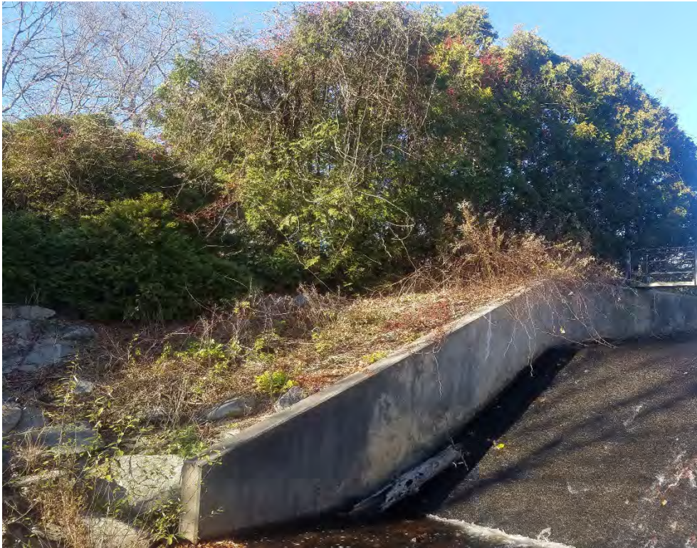
Photo 21a – Tree and brush cover along the right side abutment of the dam. See discussion under Recommendations for removal directives.
