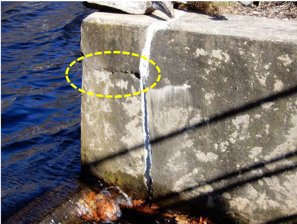
Photo 21d – A horizontal crack / joint area that needs to be monitored, adjacent to a previously sealed crack.
