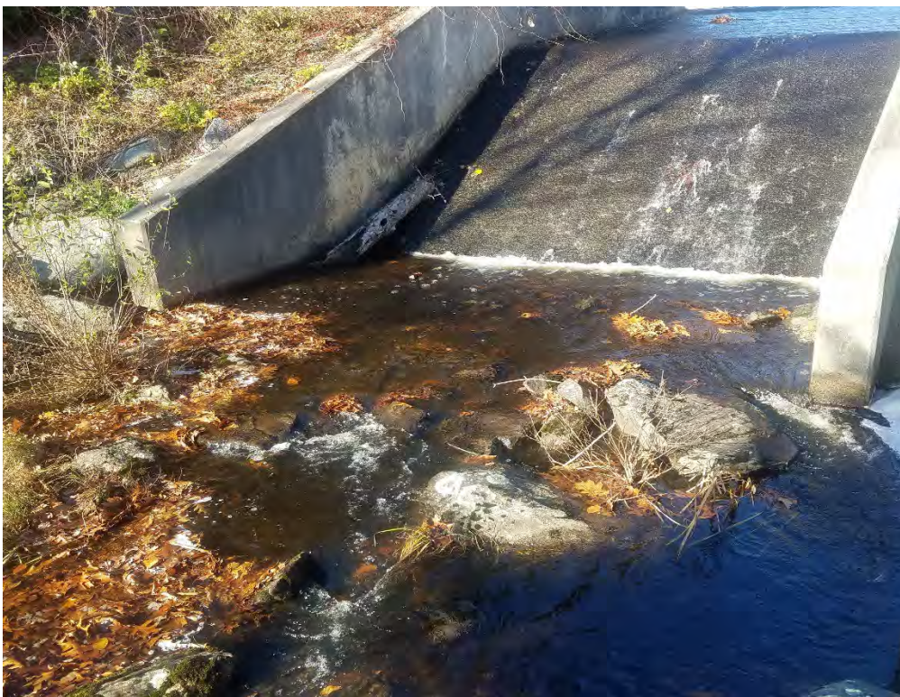
Photo 14a – The spillway stilling basin as seen from the left downstream toe.
