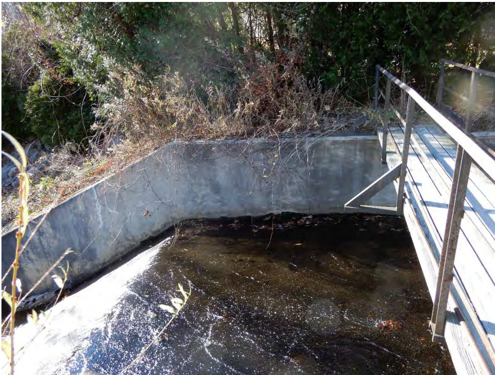
Photo 11b – The midway portion of the right side spillway training wall.
