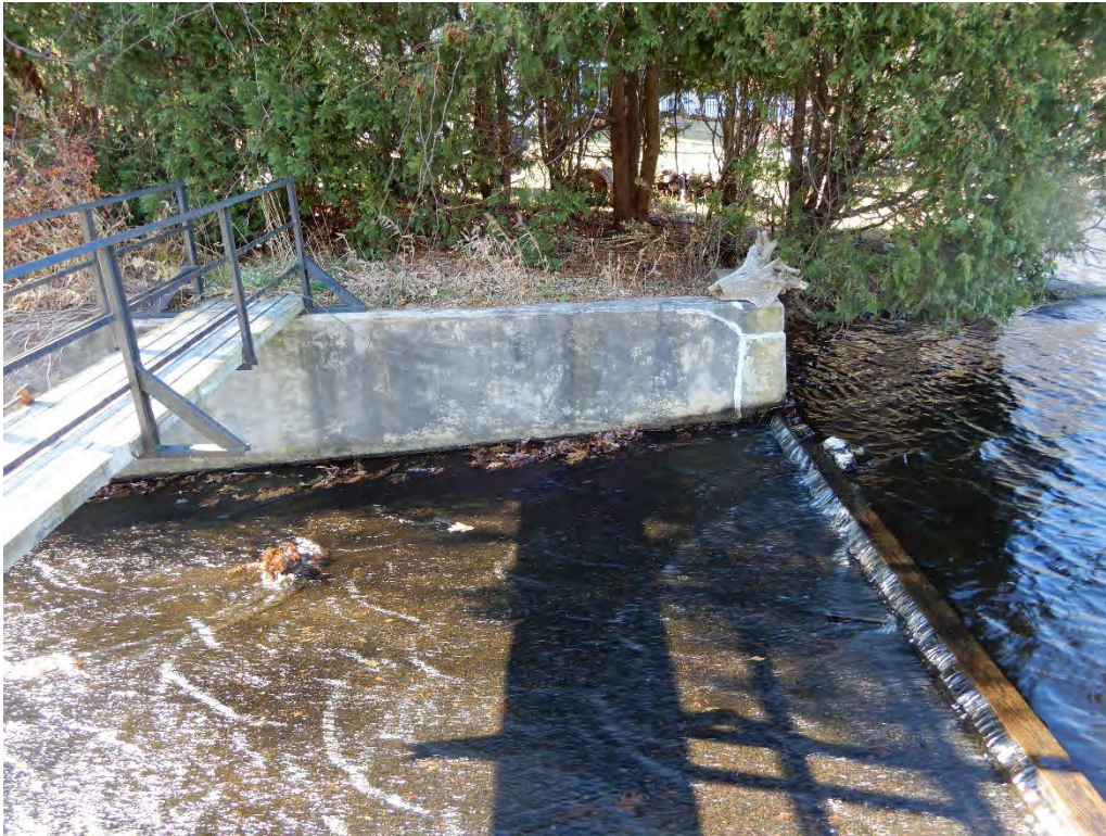
Photo 11a – The upper portion of the right side spillway training wall.
