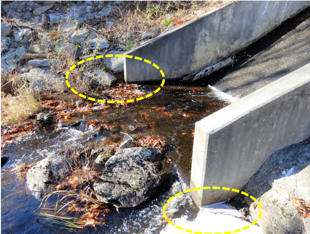
Photo 21e – Two discharge points that need to be kept clear and monitored on a regular basis. See also discussion under Recommendations.
