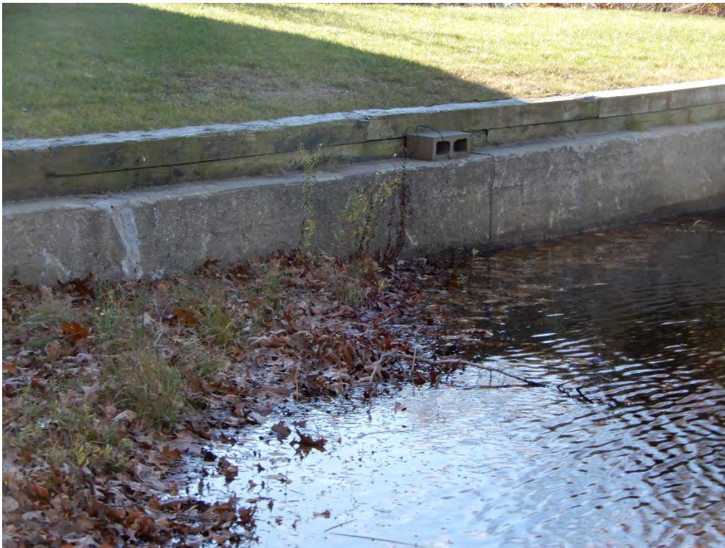
Photo 21b – An upstream area of the wall face along the left embankment where minor surficial cracking and joints were noted. Regular or routine monitoring is recommended in these areas.
